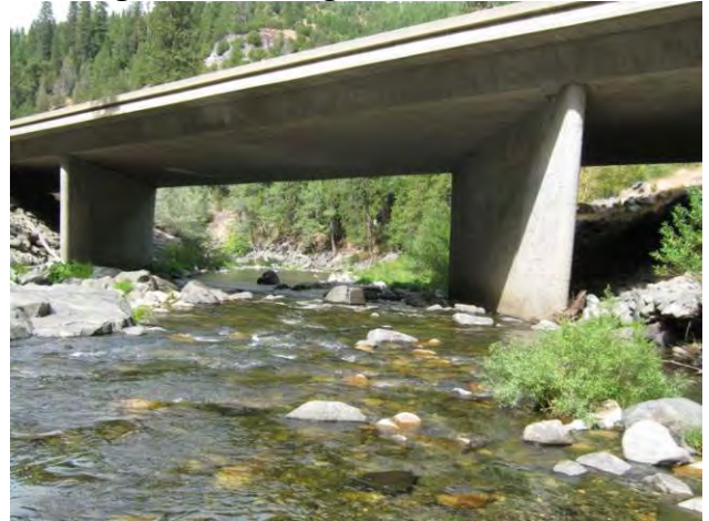
Looking N under bridge
