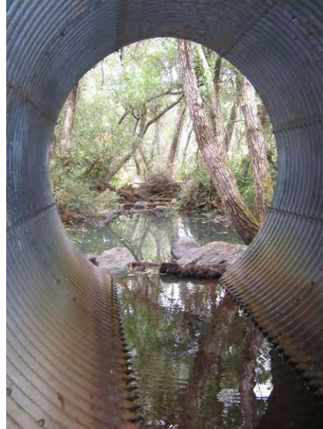
Inside culvert looking North
