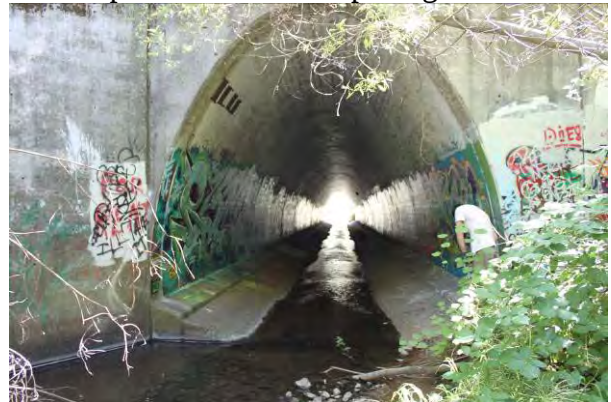
Close-up view of culvert opening
