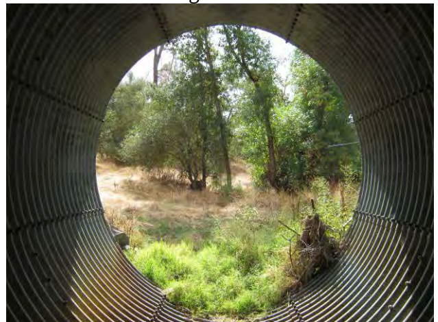
Inside culvert looking South
