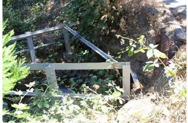
Close-up view North side
