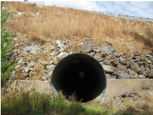
Looking North toward culvert
